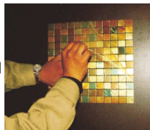
Remove the surface protective film after everything completed.
