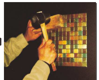
Knock the surface of Mosaic gently with a plastic hammer, a crosatie is necessary between the hammer and Mosaic.
